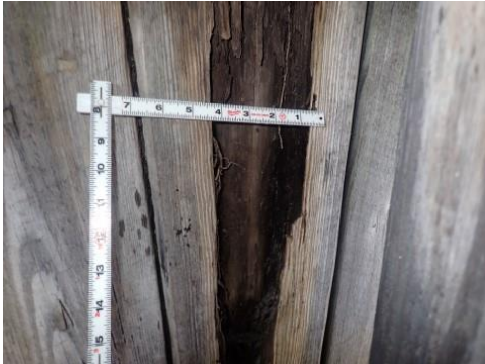
8395 - Timber Abutment Slope Protection
