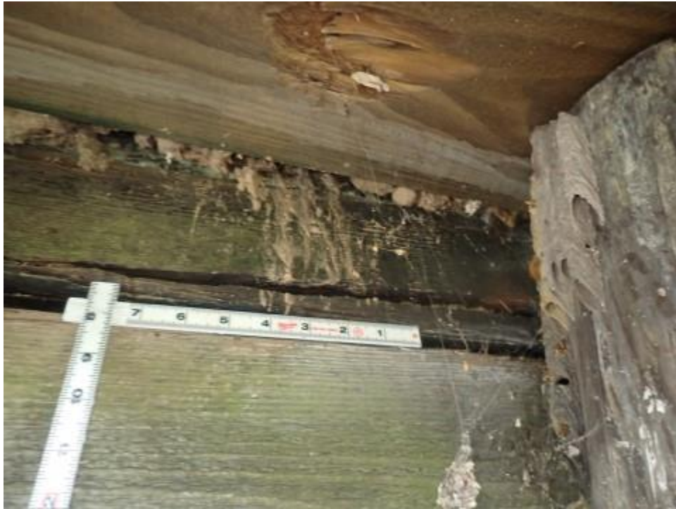
8395 - Timber Abutment Slope Protection
