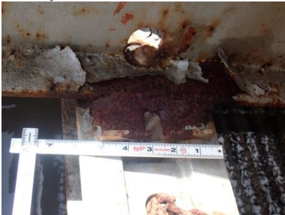
120 - Steel Truss / 152 - Steel Floor Beam
