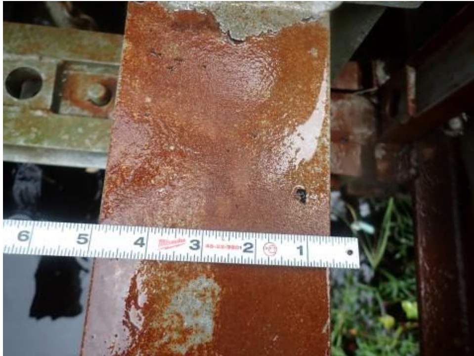
152 - Steel Floor Beam (8516 - Painted Steel)
