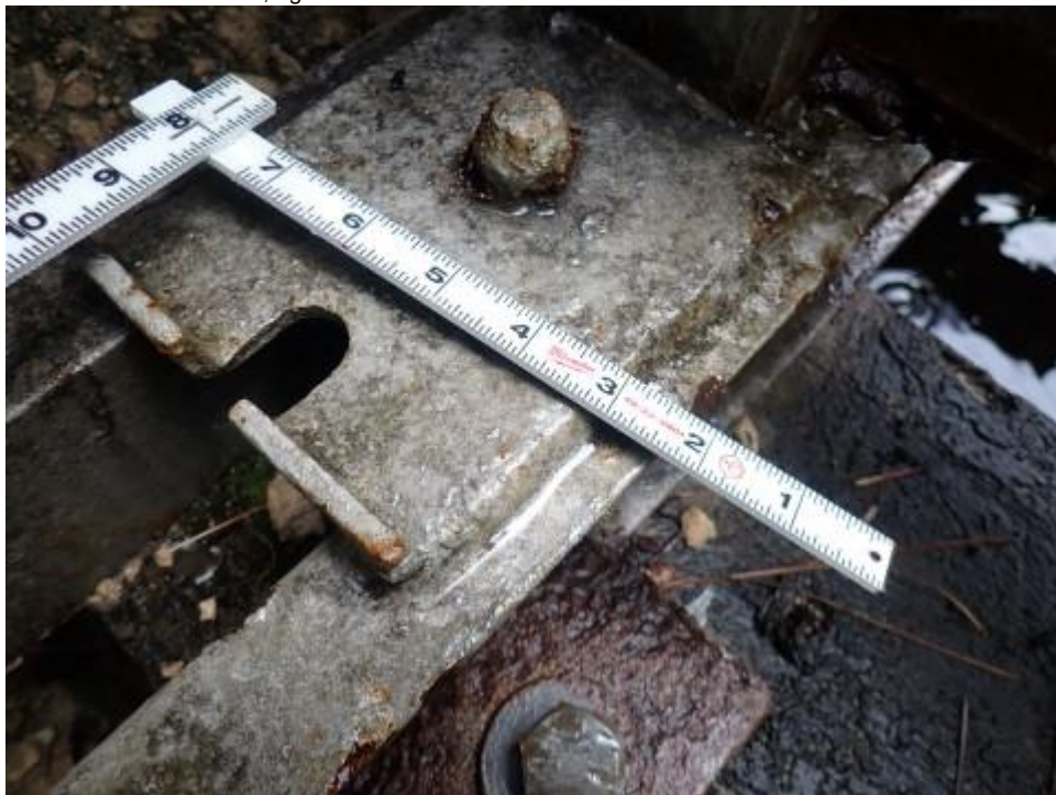
120 - Steel Truss / 152 - Steel Floor Beam
