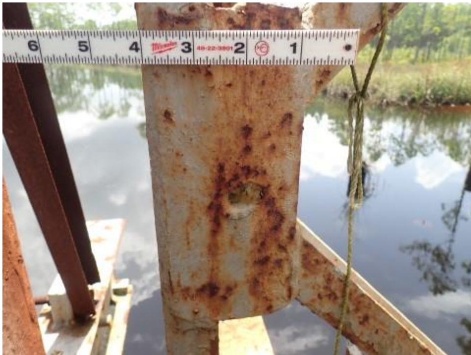
120 - Steel Truss (8516 - Painted Steel)
