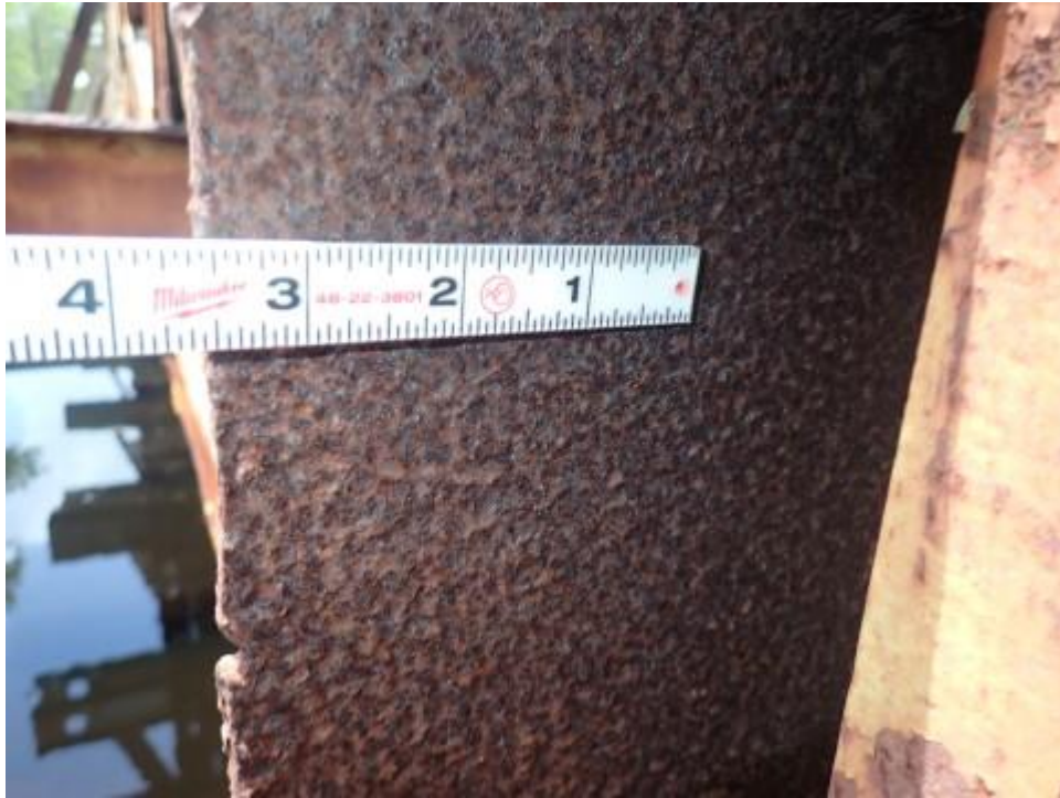
152 - Steel Floor Beam (8516 - Painted Steel)
