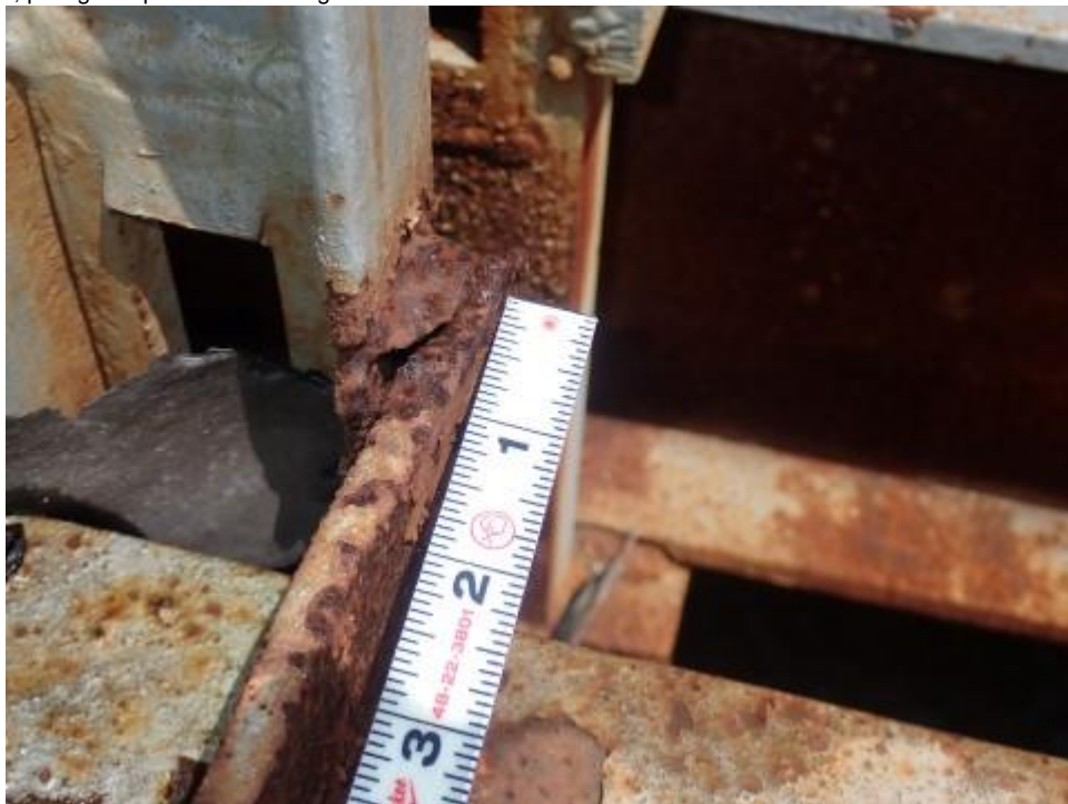
152 - Steel Floor Beam
