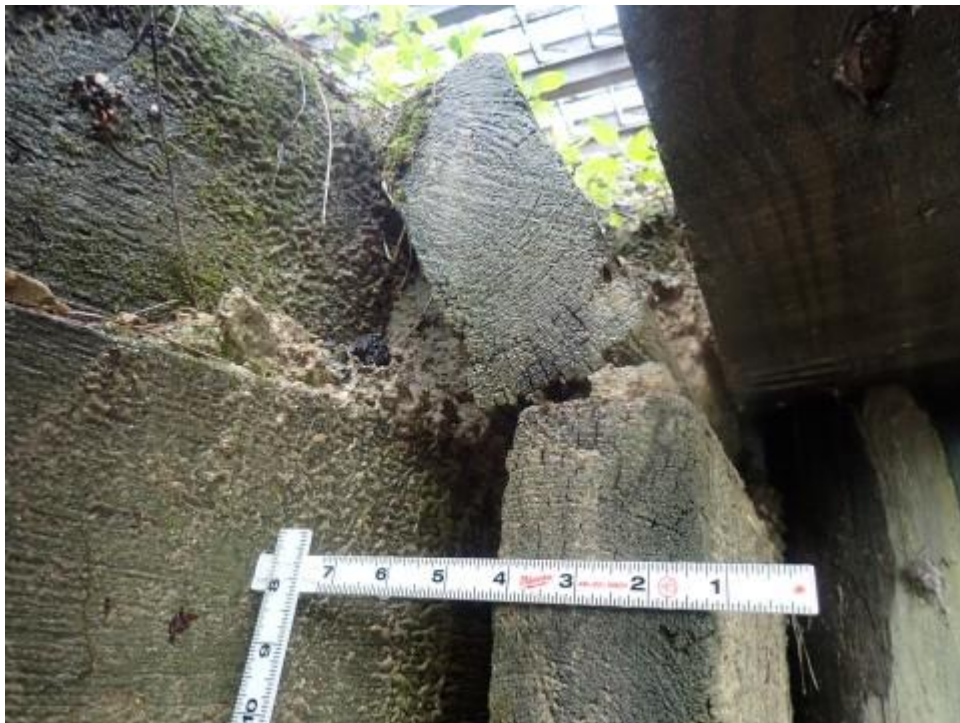
8395 - Timber Abutment Slope Protection
