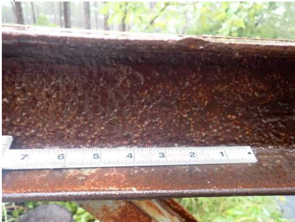
120 - Steel Truss (8516 - Painted Steel)
