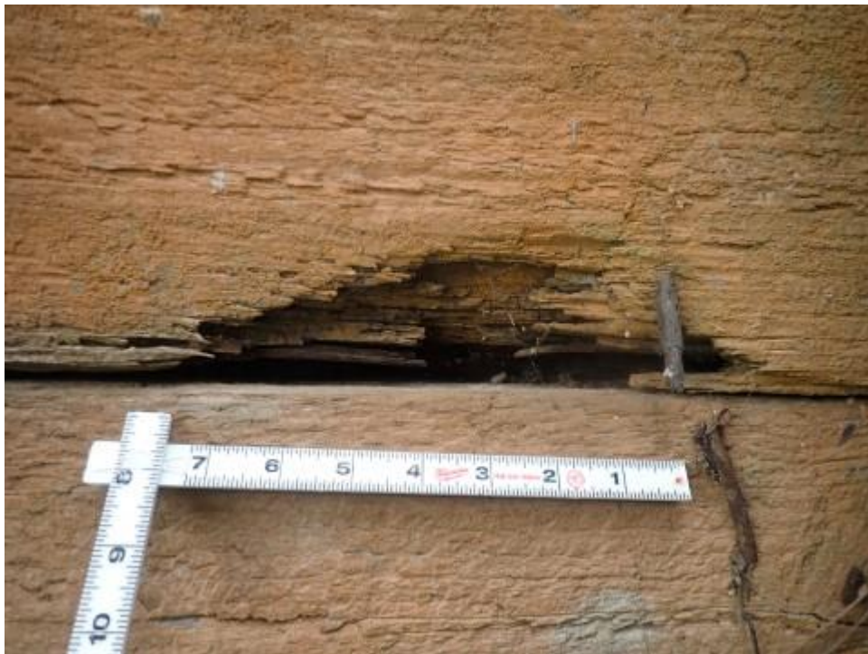
8395 - Timber Abutment Slope Protection
