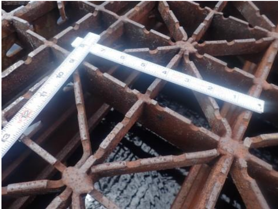
28 - Steel Deck - Open Grid (8516 - Painted Steel)
