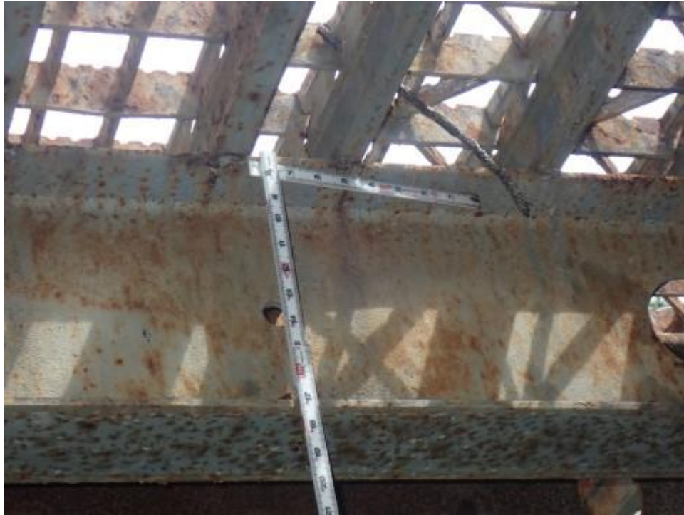
152 - Steel Floor Beam
