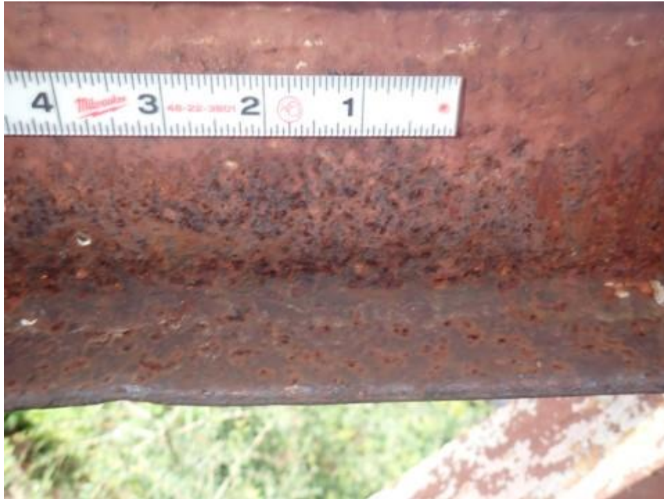
120 - Steel Truss (8516 - Painted Steel)
