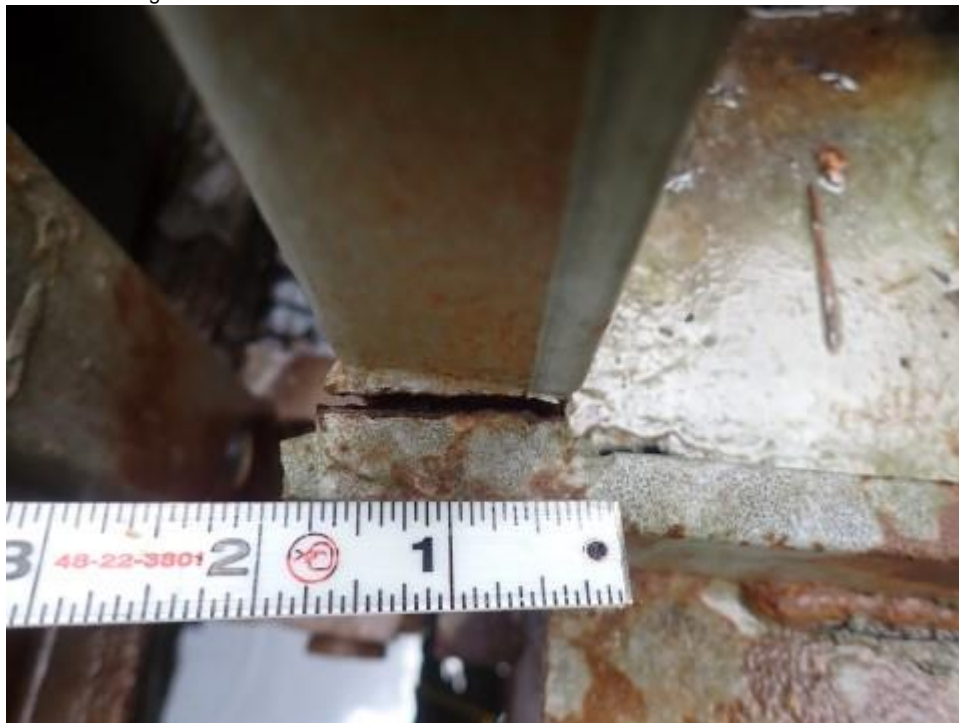
152 - Steel Floor Beam
